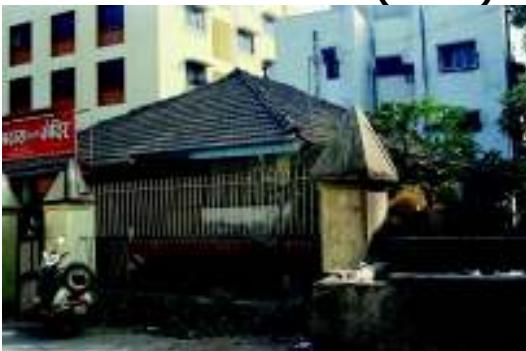
Exterior with current context
