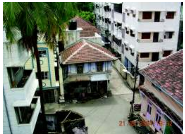
Drastic alteration of the skyline near Tungekar Rd
