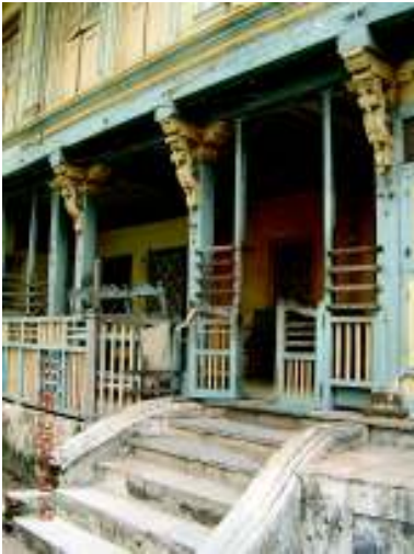
Detail of the verandah
