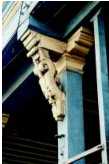
Detail of timber column and bracket
