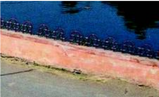
Detail of bund wall and railing
