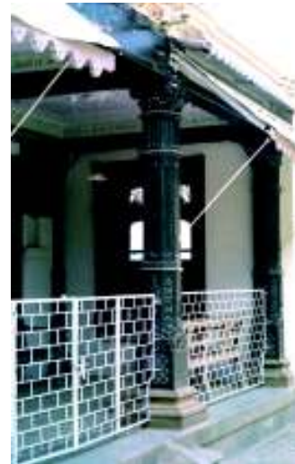
Detail of front verandah
