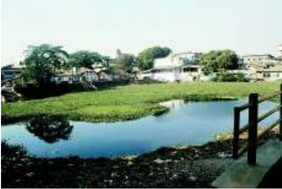
Condition of water
