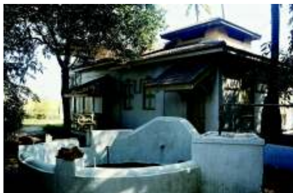
Side view showing timber roof and porches
