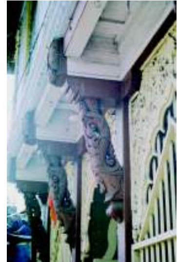
Detail of wooden brackets
