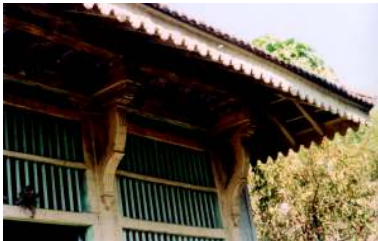
Detail of the brackets supporting roof overhang
