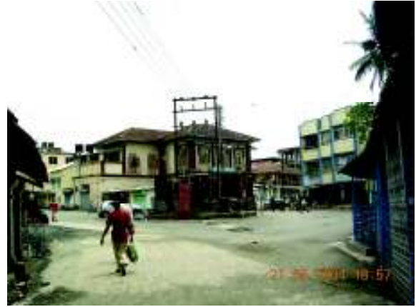
View of Zakir Husain Chowk, looking at Hawabibi Hospital
