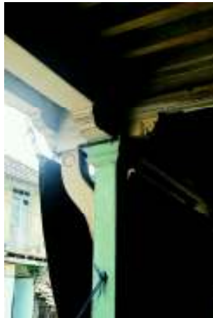
Mookri House, details of timber column and bracket in the front verandah and internal staircase
