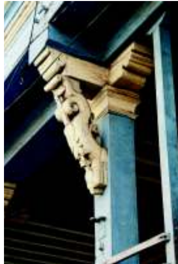
Detail of timber column and bracket
