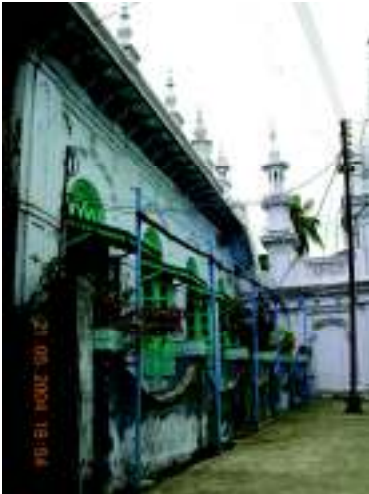
Exterior View of the Prayer Hall
