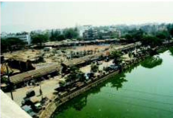
Exhibition ground on the east, where a multi-storey complex is coming up
