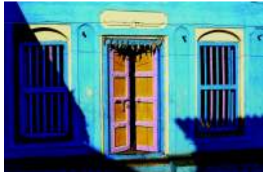
Fenestration, wooden pegs on the facade
