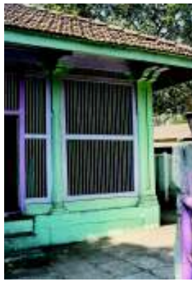
Timber frames and iron grills infills
