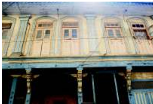
View of the pilastered bays on the upper floor
