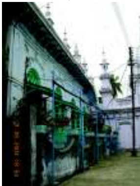
Exterior View of the Prayer Hall
