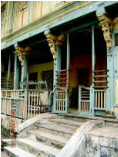
Detail of the verandah
