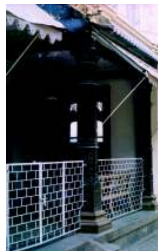
Detail of front verandah
