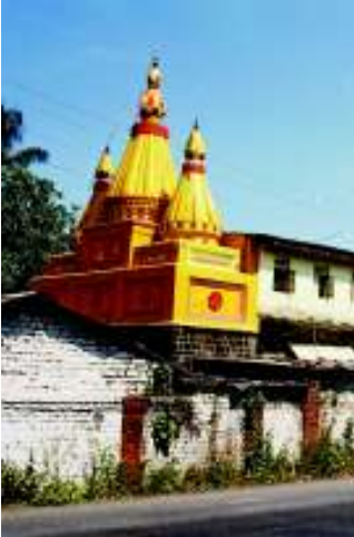
Exterior view from Panvel-Uran Road
