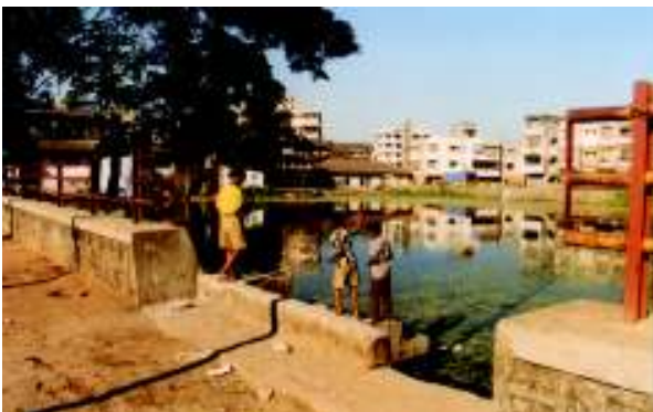
Bund wall, railing and steps
