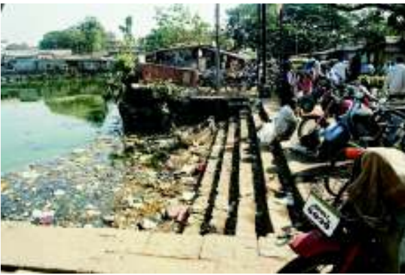
Condition of the steps
