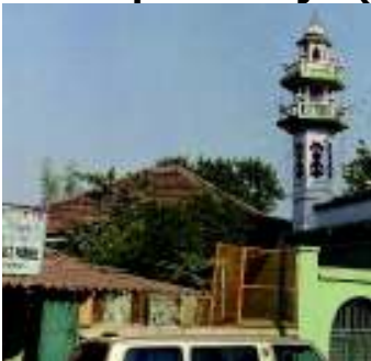
Exterior with hipped roof
